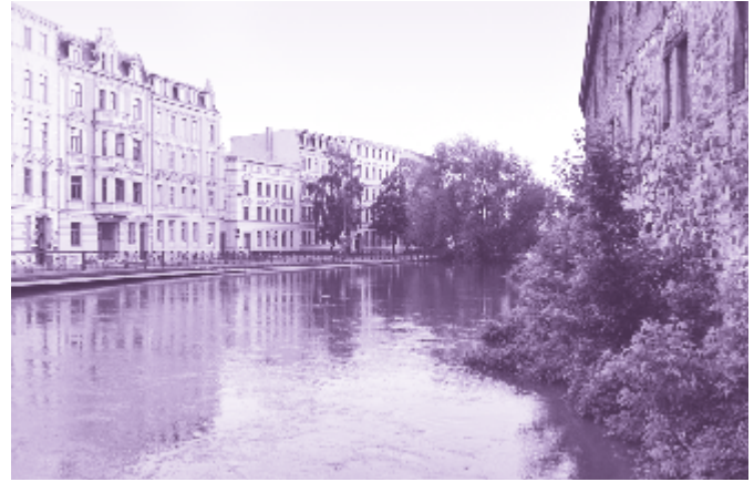
Improved flood protection needed: flooded streets in Halle (Saale) in June 2013.
