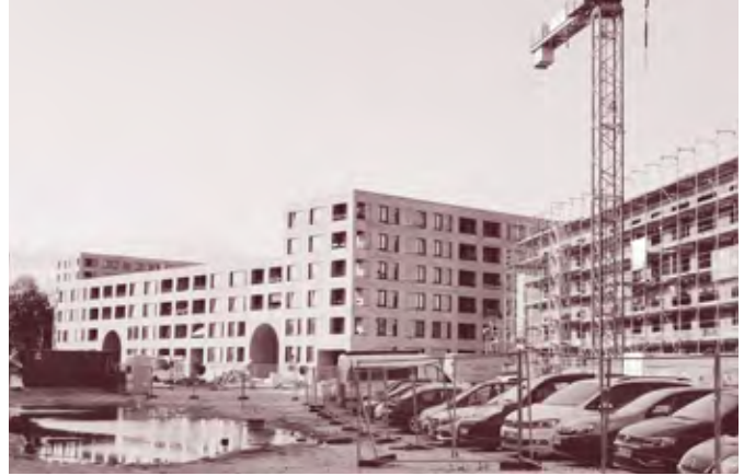
In Hamburg North, most garden lots had to make way for office complexes.
